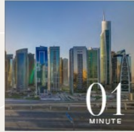
Jumeirah Lakes Towers
