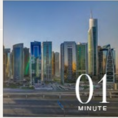
Jumeirah Lakes Towers
